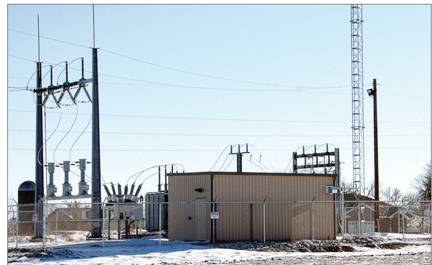
Hallberg. In the middle is the Clark Wind Farm substation located north of Clark. Power from the wind turbines interconnects with the NorthWestern Energy line. The Clark Wind Farm will light over 5,000 homes. The power goes west from Clark.
