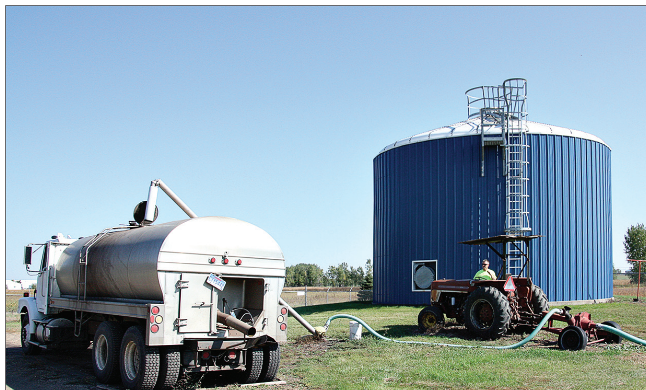
This time of year is a very busy time for city employee Darin Altfillisch. The water/sewer superintendent will be hauling sludge from now until freeze up. Sludge is stored in the big blue tank and pumped to the sludge truck. It then is placed on area fields.
