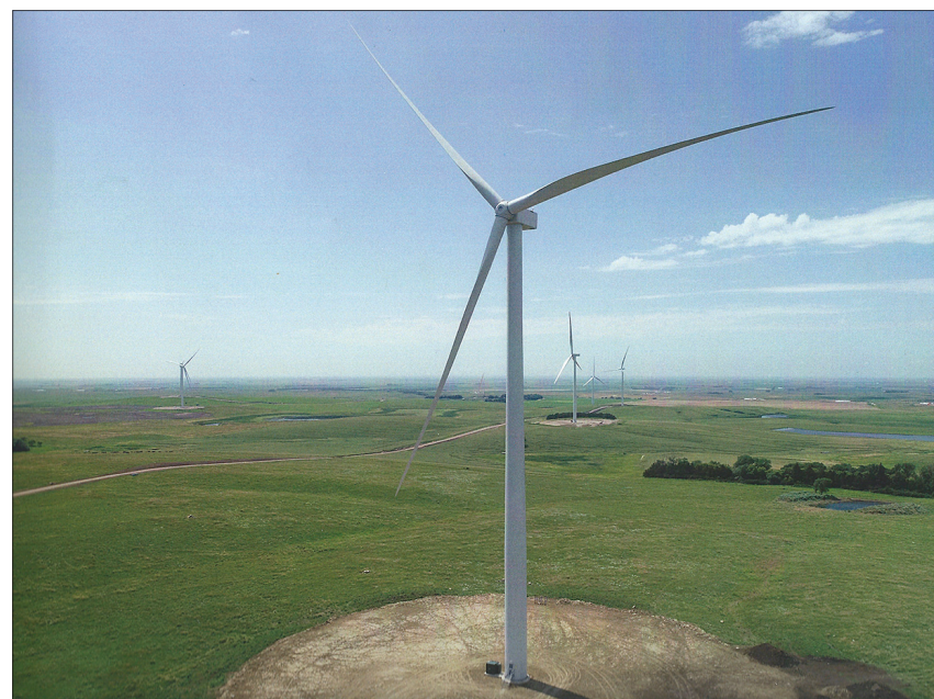
Arguably the top story in 2019 in Clark County is the construction and completion of the Geronimo Energy Crocker Wind Farm. Geronimo Energy has now sold the energy to Walmart and Cargill. The wind towers are now turned on. This photo was taken on August 13.
