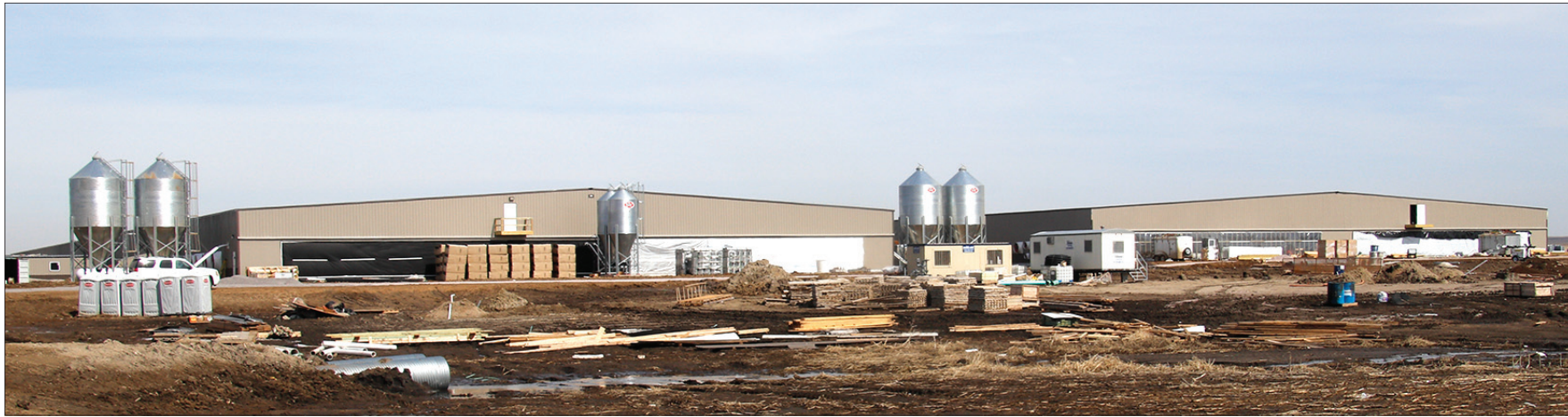
Located near the intersection of 417th Avenue and 178th Street in Clark County is the newly finished Husky Farms operation, a breed to wean hog farm.
