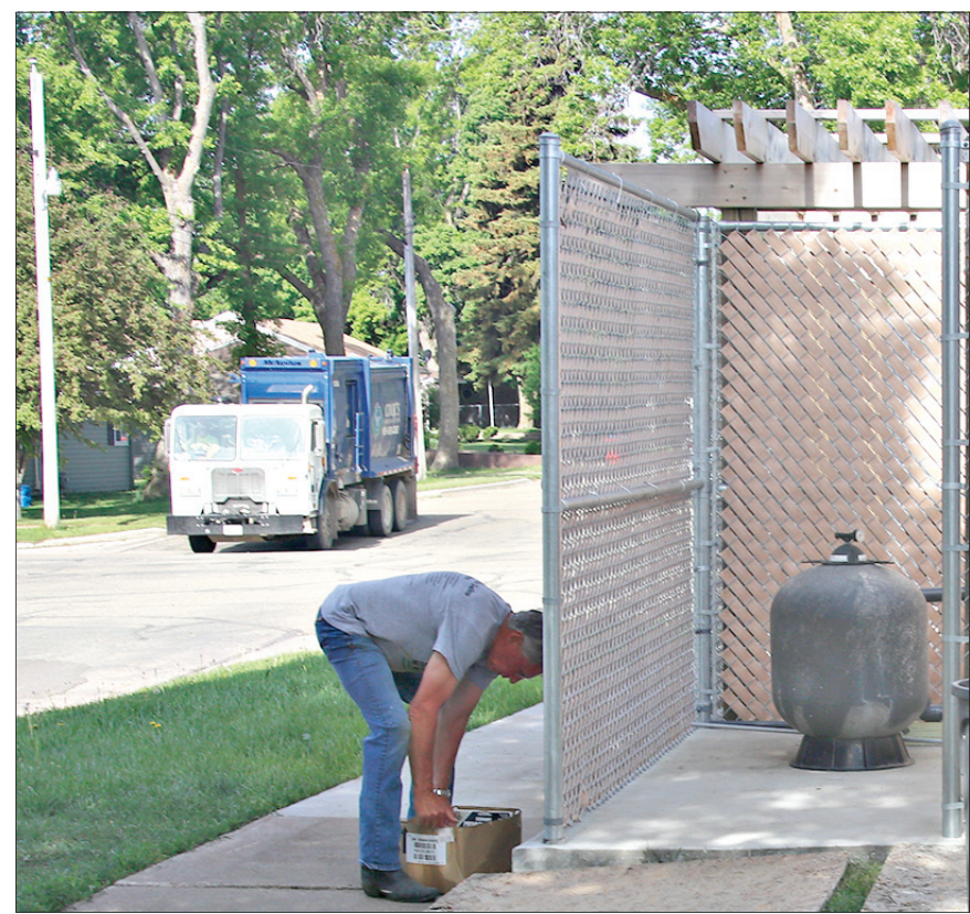
This is the pump area next to the new splash pool - at the Clark Horace Bennett Memorial swimming pool. Weaving a vinyl type of ribbon through the fence adds some shade and cover to the area. The weaving continues over to the pergola area at the kiddie pool/splash pool. Harvey Spieker finishes for the morning as he has spent a lot of volunteer hours this spring working at the pool site along with city councilman Brian Cook.
