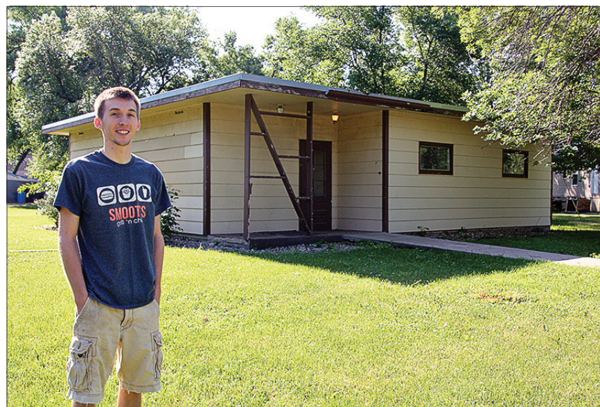
Wyatt Warkenthien, (a 2012 WLHS graduate) purchased the former senior citizens building at 302 Lincoln Avenue in Willow Lake, last October. Along with family members Kerry and Paula Warkenthien and Kurtis and Bonnie Siebrands the building has been renovated and 'upcycled' to house a tanning bed business as well as being available for family reunions, birthday parties, showers, graduation receptions and similar gatherings. Wyatt's family also makes their unique wooden sandboxes and tables at this location.
