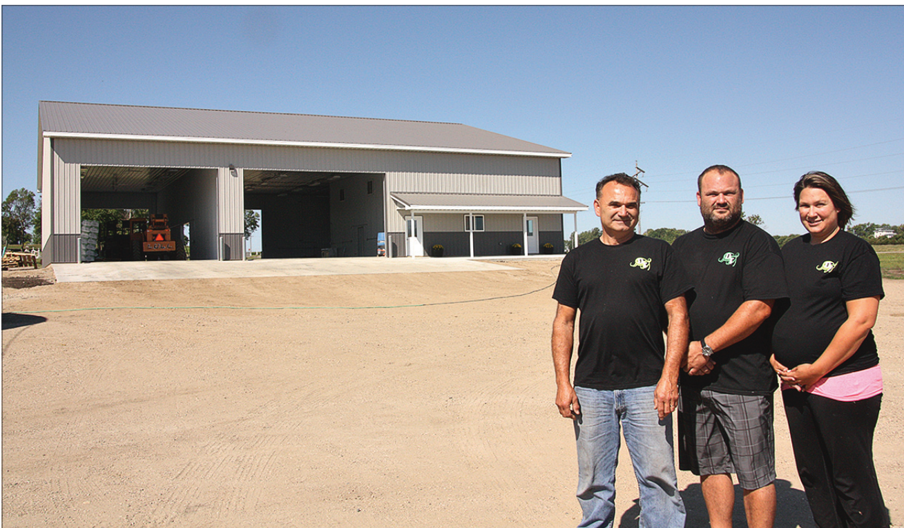
Duenwald Transportation has basically outgrown its former bus garage so a new one was in order and is close to being completed. With an open house planned for mid October, if construction goes as planned, Duenwald Transportation, its offices, Dan's
